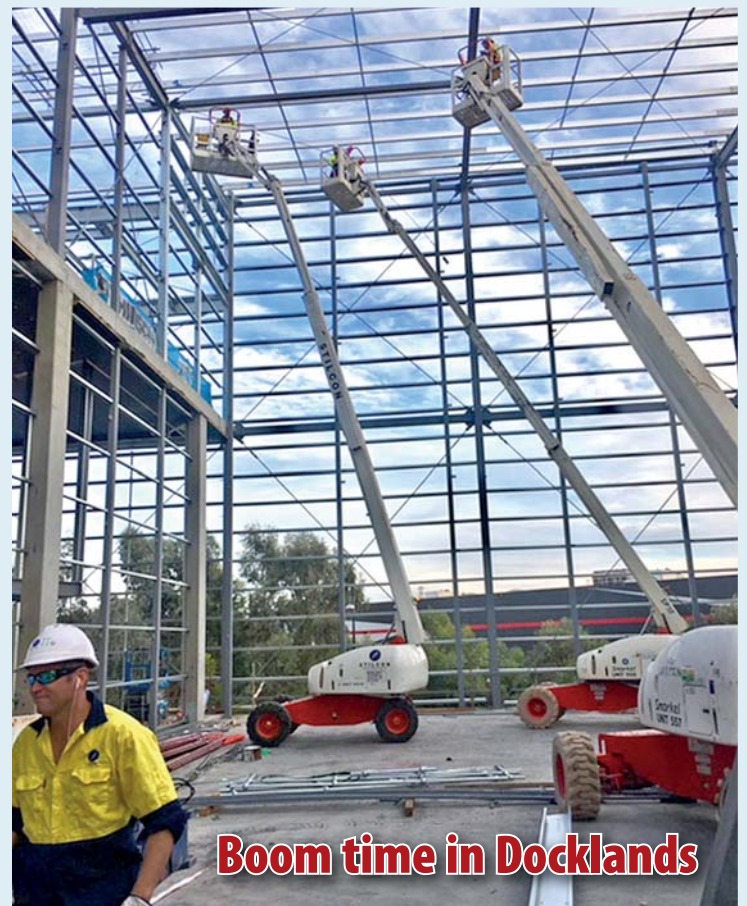
Harbour Town Cinemas in Docklands, Melbourne, are taking shape. Hutchies' project was given a helping hand recently by steel contractor, Stilcon, who had three booms working simultaneously at a height of 15m.
