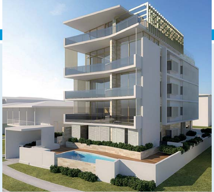
A five-storey beachside apartment building is under construction at Miami on the Gold Coast.
