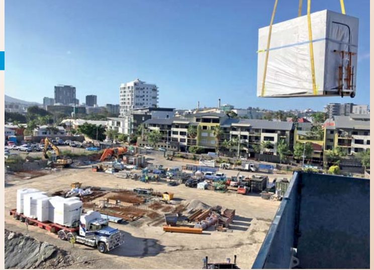
Pods being delivered on site.
