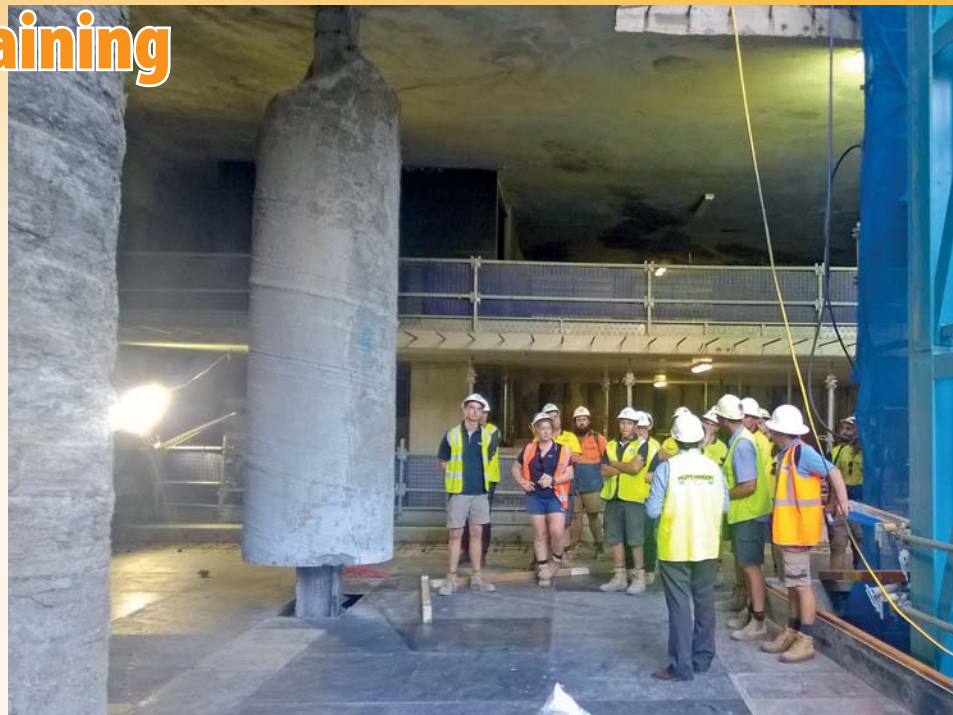
Apprentices on site learning about top-down construction.
