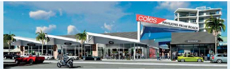
Hutchies is undertaking an extensive revamp of the Pavilions Shopping Centre in Palm Beach on the Gold Coast.
