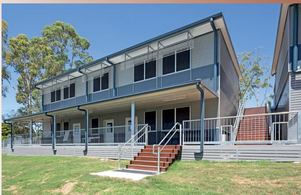
Modular classrooms at Mansfield State School mark the latest roll-out in a four-year supply agreement for schools across Queensland. Mansfield is also noted as the high school attended by all the members of the band, Violent Soho.
